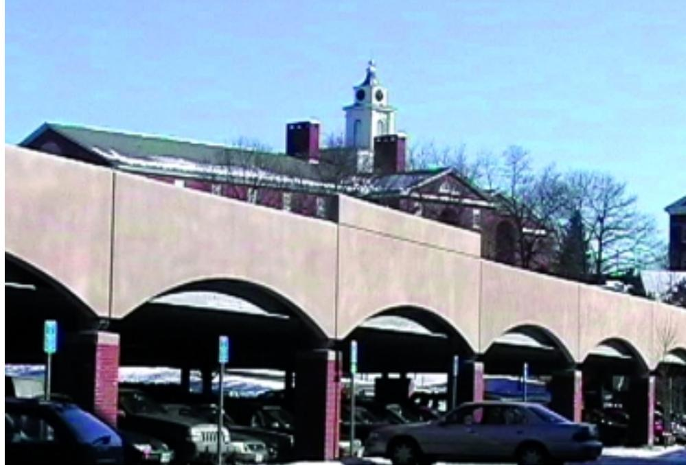
Parking had to be built quickly during the summer “slow down” since the structures were being constructed over existing surface lots. Prime Steel erected the entire parking structure, including precast concrete façade spandrels, in one week. Masonry piers and mechanical systems were installed after erection allowing for the parking structure to open concurrently with the renovated dormitory for first-year student orientation on campus.
