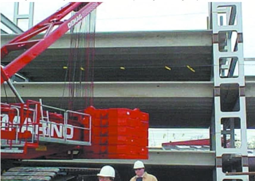
The Yale University School of Medicine parking structure under construction. Note the use of Hybrid Parking Solutions' prefabricated double-column sections to support precast concrete tees.
